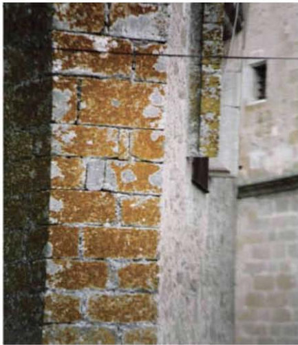
Figure 3. Patinas aspect in granite and their colour of cut-water (Northwest façade of bridge at Cáceres).
