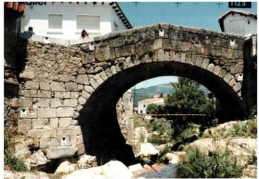
Figure 4. Granite bridge at Cáceres (East facade).
