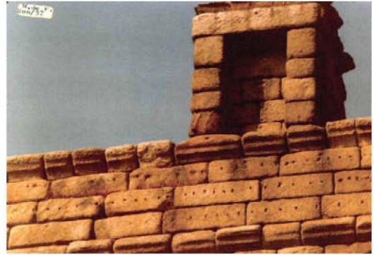
Figure 2. Natural orange colour of the granite (East façade of aqueduct at Segovia).
