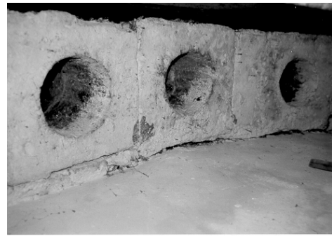
Fig. 6. See in photograph the wedgestones of the old built-in arch where the bathtub has been introduced.
