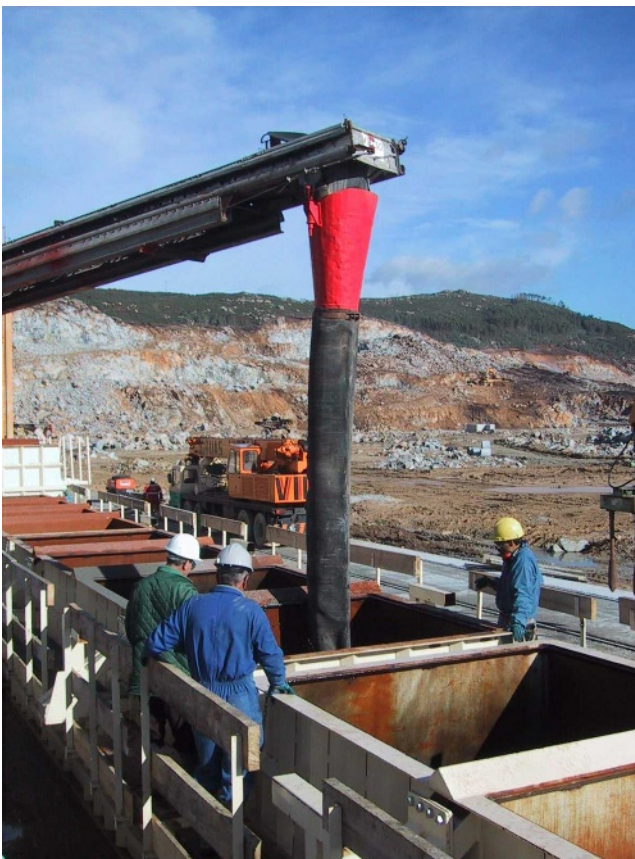
Figure 11. Close-up of the distributor arm or 'crawler'
