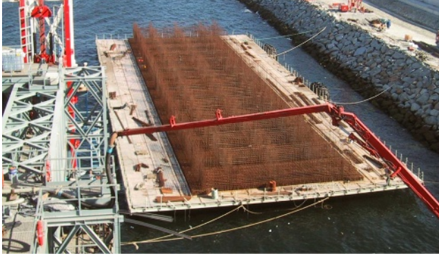
Figure 18. Preparing the footing for the wharf caissons
