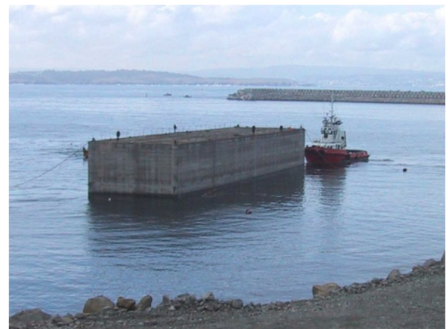
Figure 17. Close-up of the caisson laying process
