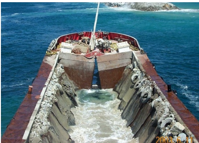
Figure 5. Depositing the riprap on the seabed
