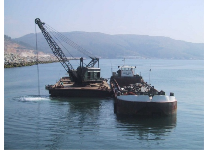
Figure 16. Extracting material dredged in rock
