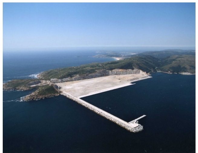
Figure 20. Final state of the works, August 2004
