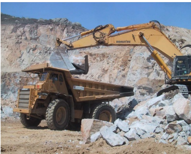
Figure 2. Equipment used for loading and transporting material
