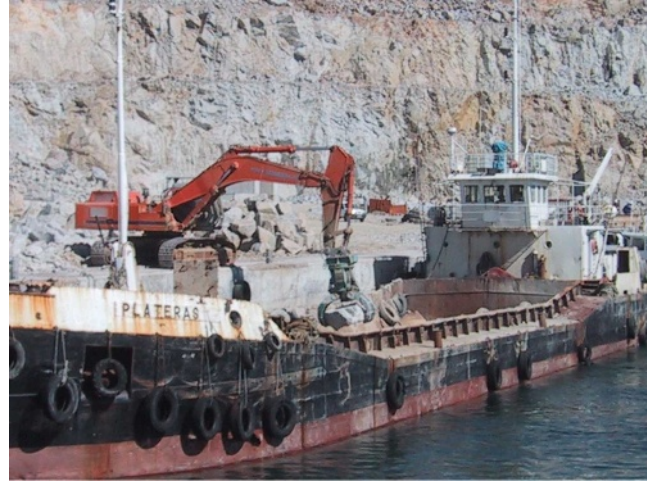
Figure 6. Loading a barge with a back digger from the auxiliary quay
