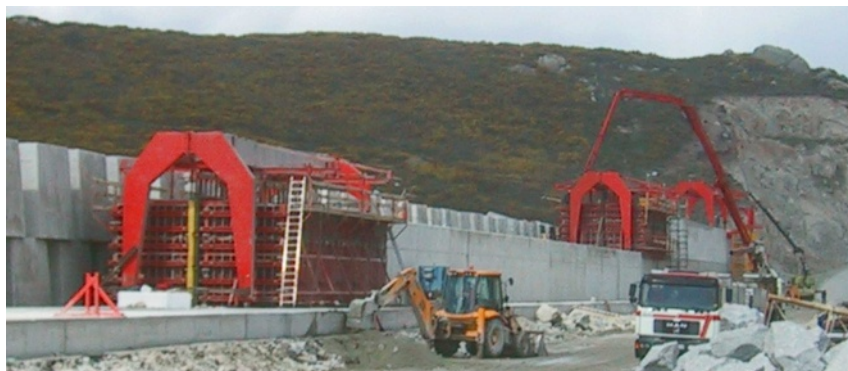
Figure 14. Close-up of how the parapet construction work was progressing
