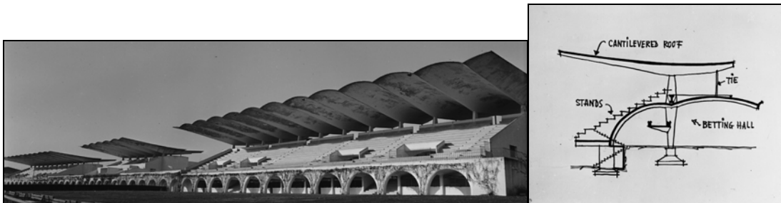
Figure 1. Panoramic photograph of the decks and construction scheme.
