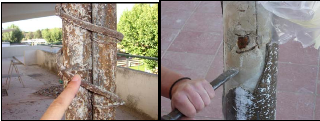
Figure 8. Ties restoration.
