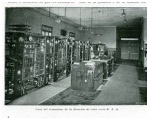
Figure 4. Aranjuez EAQ transmitter equipment
