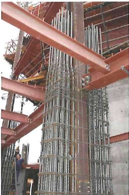
△ Figure 3 Torre Sacyr-Vallehermoso: composite column before concreting
