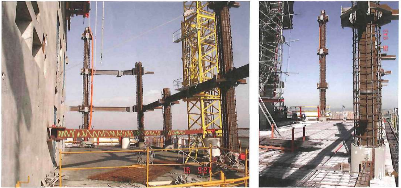
△ Figure 5 Torre de Cristal: assembly of the composite columns
