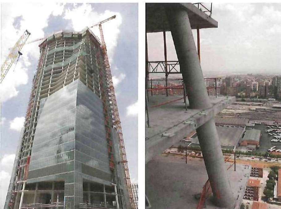
△ Figure 8 Torre Espacio: inclined columns that disappear in the upper floors
