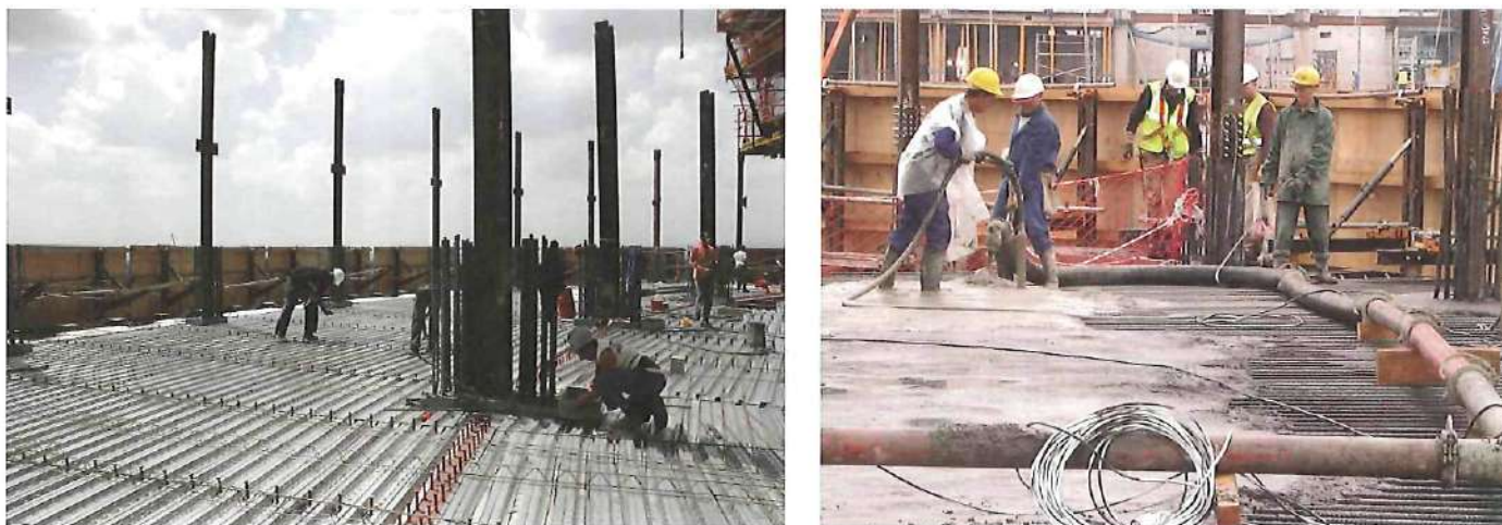
△ Figure 9 Torre Sacyr-Vallehermoso: assembly and concreting of the composite slab
