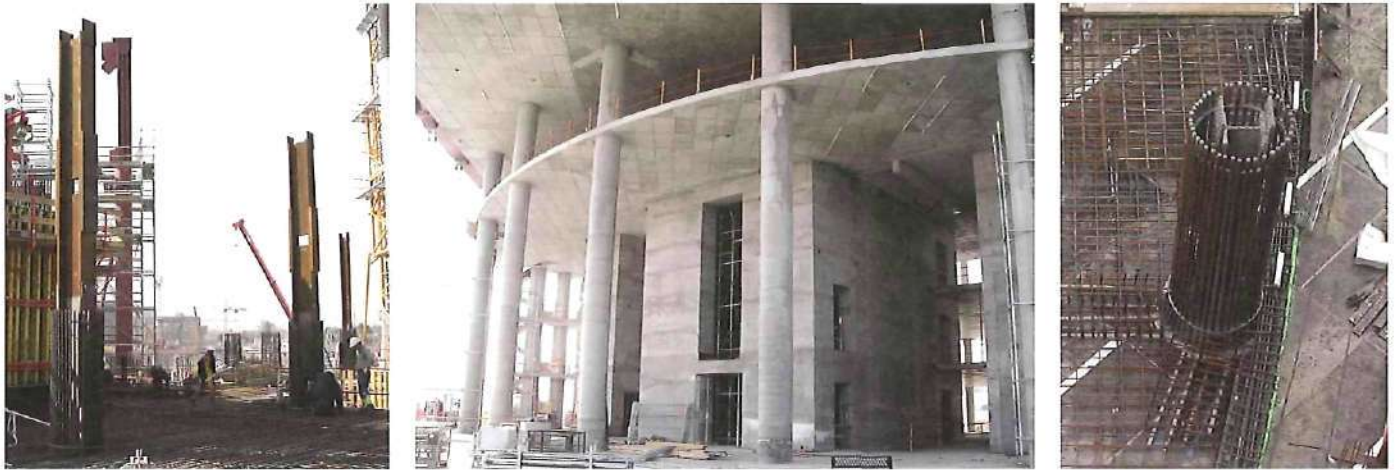
△ Figure 7 Torre Espacio: composite columns at the base of the tower
