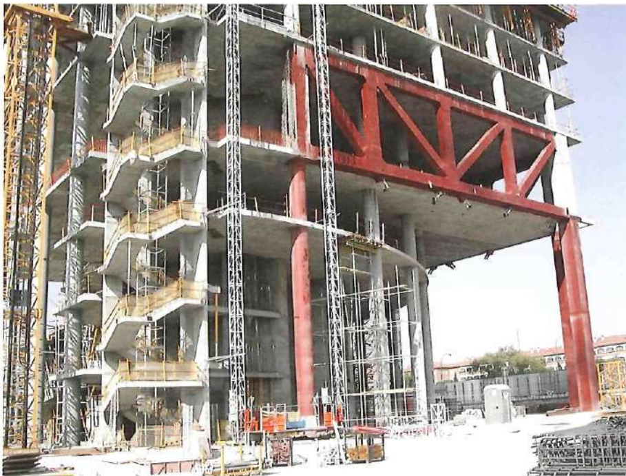
△ Figure 17 Torre Espacio: composite trusses at the base of the tower
