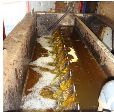
Fig. 3 Sewage treatment plant
