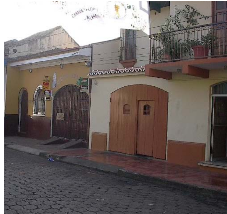
Concrete, 2 stores, after 1972
