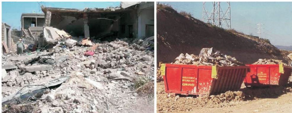
Fig. 3: Demolition works waste. La Rozas, Madrid autonomous community. (June 2007).
