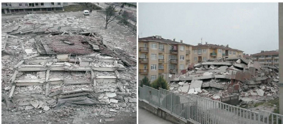
Fig. 1: Demolition works. Majadahonda, Madrid autonomous community (June 2007).
