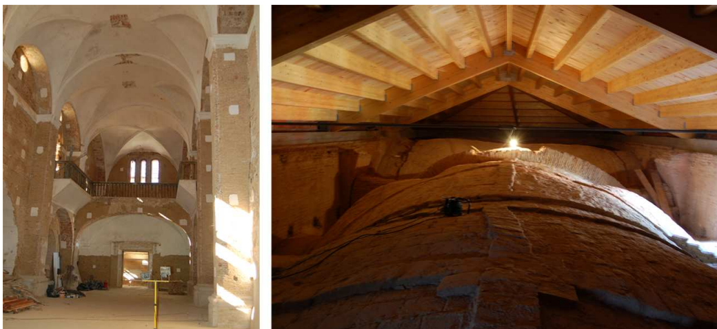
Figure 2: (a) internal view of the nave; (b) extrados of the vaults over the nave
