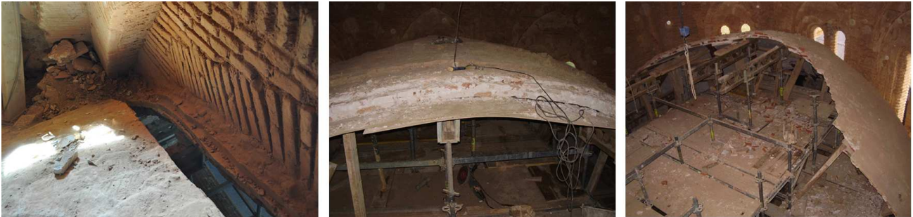
Figure 6: Sequence of the demolition of the vault.
