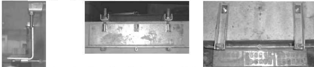
Figure 4 a) Side view of Halfen-AllWall Pi-Bracket with its vertical (Z) and horizontal (Y) adjustments; b) Frontal view; c) View of bracket supporting the first brick in the lintel course.
