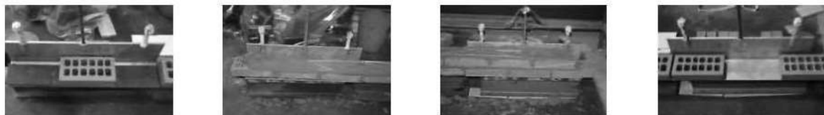
Figure 13. Left support of the lintel with neoprene layer between brick and steel.
