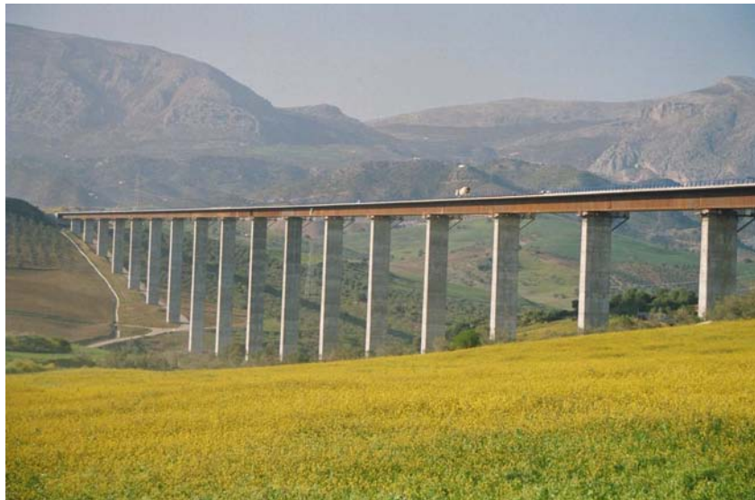
Figure 1. Viaduct “Arroyo las Piedras” for the HSR line Córdoba-Málaga, Spain (2007). Continuous deck of length 1209 m, spans of 63,5 m and piers taller than 94 m.
