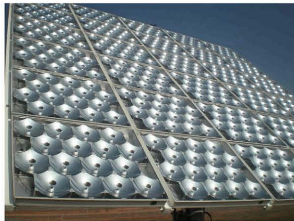
Figure 10 (online colour at: www.pss-a.com ) Top: Concentrator photovoltaic (CPV) systems of the company Concentrix Solar GmbH installed at the ISFOC. Bottom: CPV modules of the company Solfocus Inc all installed at the ISFOC (photo courtesy: ISFOC)
