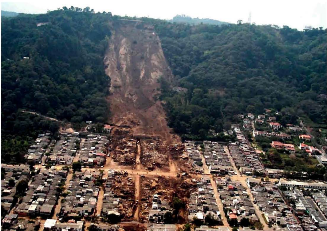
Fig. 3. Aerial view of the earthquake-triggered landslide in Las Colinas, El Salvador, on 13 January, 2001.
