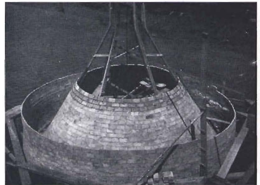
Figure 2 Foundations of Sancti Petri Bridge under construction. (Source: Torroja archive)
