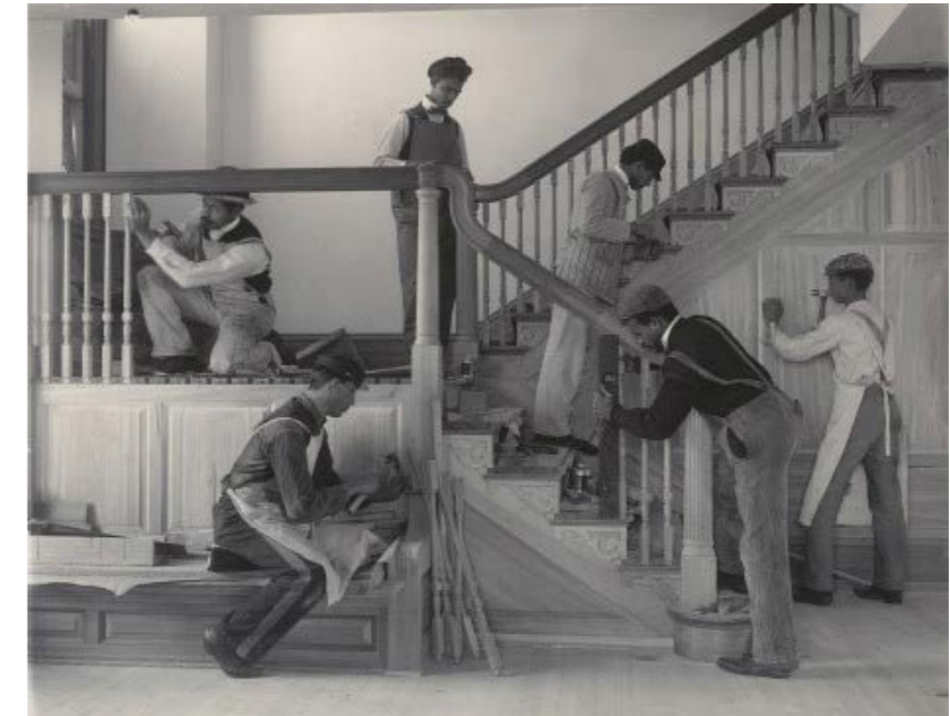
FIG. 2.1 – Stairway of the treasurer’s residence. Frances Benjamin Johnston. 1900. Fuente: MOMA
