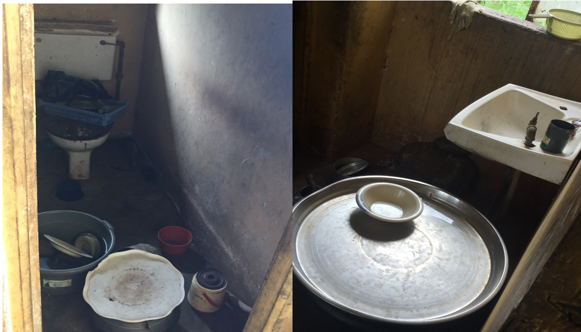
Figure 1: Picture of the dual kitchen/toilet at the Ansarudeen Primary Health Care Center, Imasayi, Yewa North Ogun State
