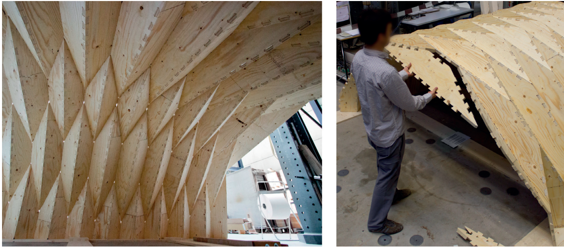
Figure 3.8 – The MTSJ joints have already been successfully applied to more complex assemblies, where the joint angles \theta_1 , \theta_2 and \theta_3 are not zero ( Robeller et al, 2014).
