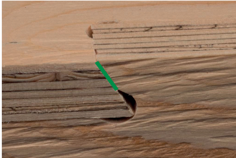
Figure 4.7 – Reduced contact on the locking faces.
