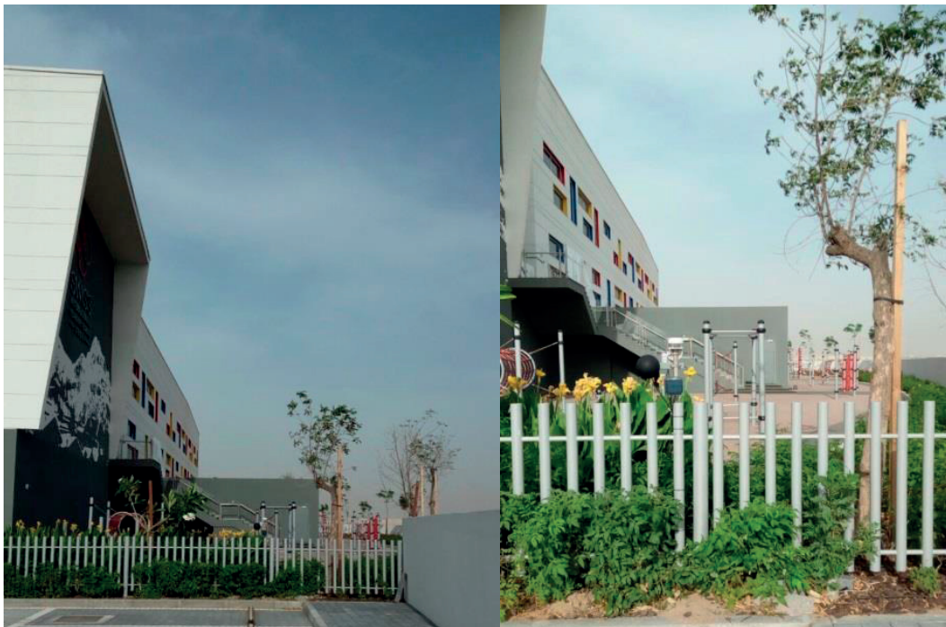
Figure 5.44 WS-1713B, located on the southern entrance of the building, near the playground area (17 th of May to the 2 nd of July). Photos by Ashfaq Khan.
