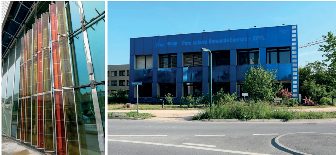
Figure 4.4 Photovoltaics panels on the EPFL campus. Gretzel cell (left) and Kromatix™ (right). Source: Mediatheque EPFL.
