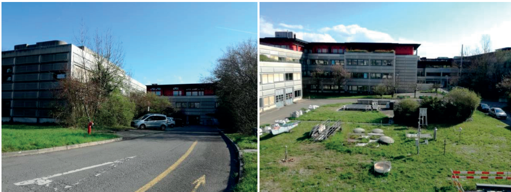
Figure B.1 PH (left) and GR building (right).
