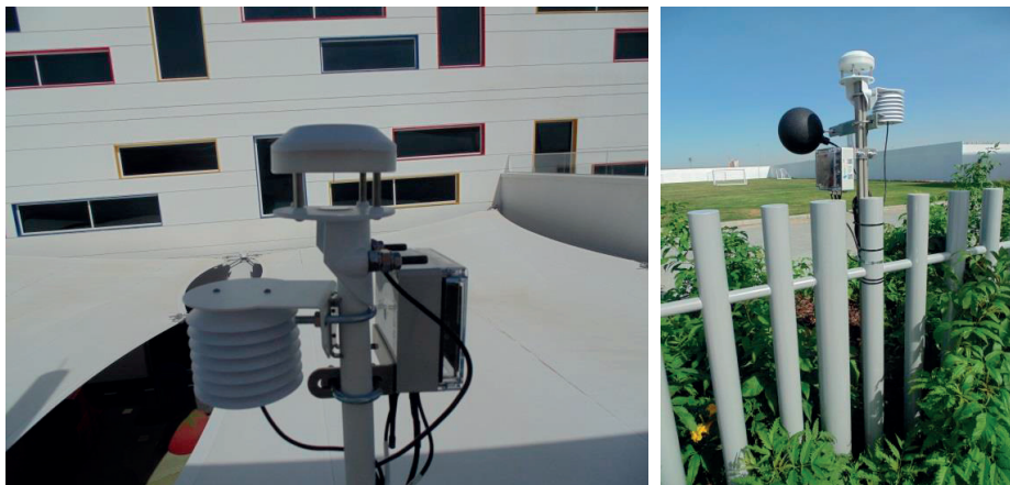
Figure 5.47 WS-1712, in the first floor playground (Left) and WS-1713A in front of the temporary football court
