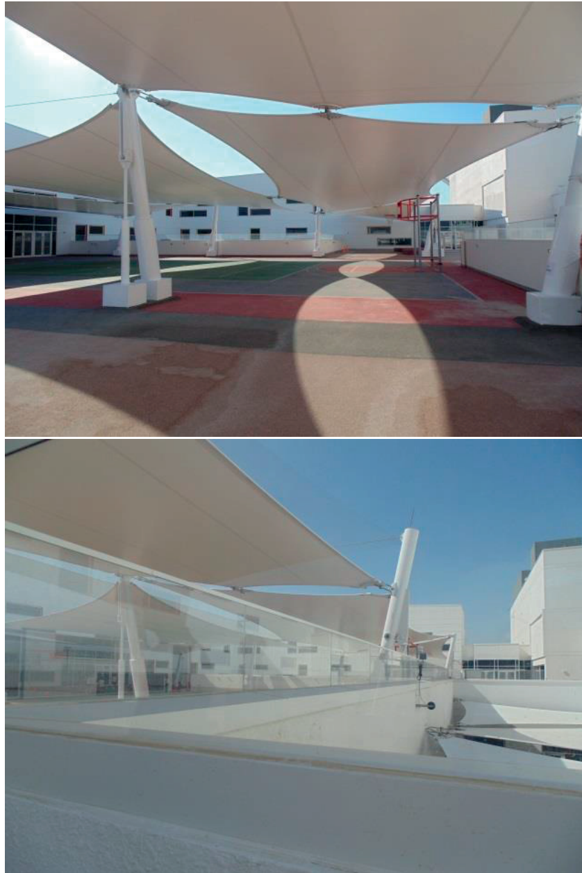
Figure 5.42 WS-1712, located on the first floor, in the playground/ sports area.
