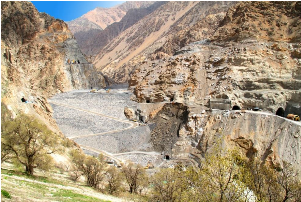
Figure 2. Rudbar Lorestan dam under construction, upstream view ( www.iwpc.ir , 2015)
