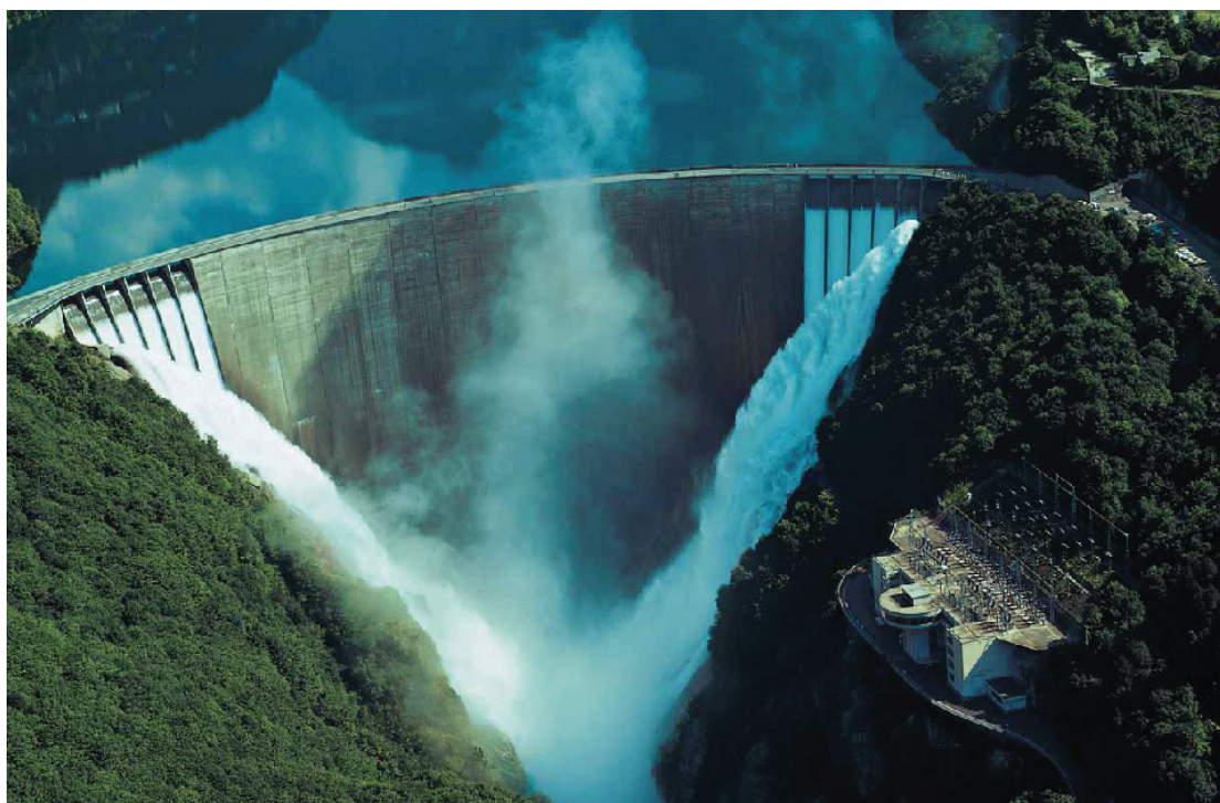
Figure 9.30: Photo of the Contra dam (SwissCOD, 2011).
