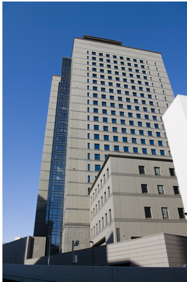
Figure 1: The NII main building.
