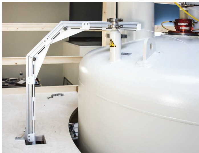
Fig. 48 A : Linear segment of 30 cm length (1), segment with a bend smaller than 45^\circ and a segment with a bend larger than 45^\circ . B: photograph of an implementation of this kind of tunnel, here the tunnel to the 800 MHz spectrometer installed at ENS Paris. C: photograph of the last part of the same tunnel.
