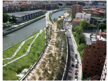
Γέφυρα Oblicuo Oblicuo bridge
