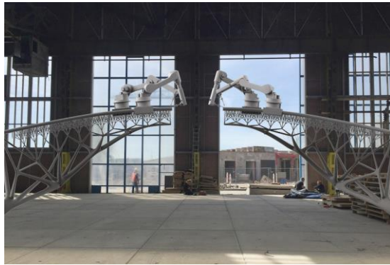
Figure 3. Robots are going to autonomously create a steel bridge [21].
