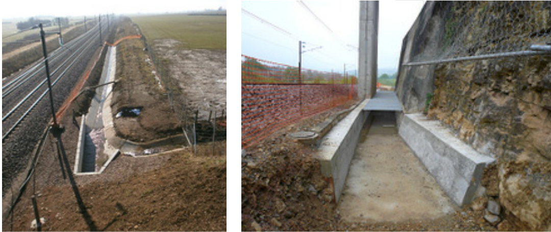
Figure 5: Pictures of rehabilitation works on the outskirts of a HSL
