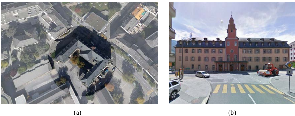
Figure 2: Top view of the building in the historical center of the city of Sion (a) and view of the building's façade (b) (Source: Map data ©2015 Google).
