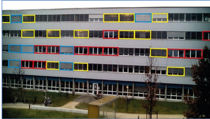
Figure 1: Photo of the west façade of building PSE-C on February 5, 2013, overcast sky
