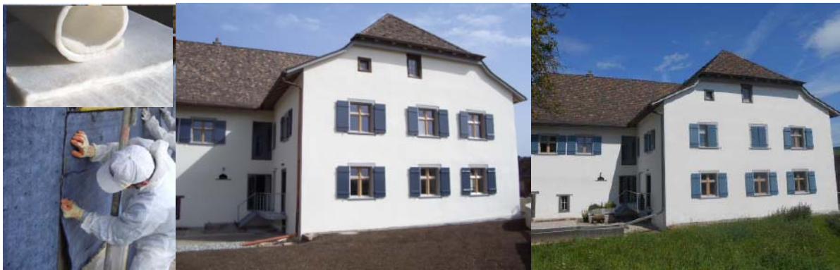
Figure 2: Aerogel sheets of 1 cm thicknesses like the old mill in Oberhallau near Schaffhausen, CH
