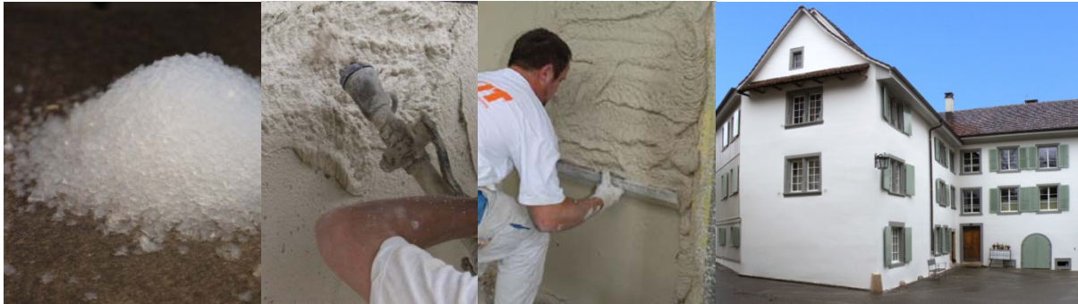
Figure 3: Aerogel granules (left) as used in the aerogel plaster (centre images), and the 2012 retrofitted old mill at Sissach near Basel, CH (left)
