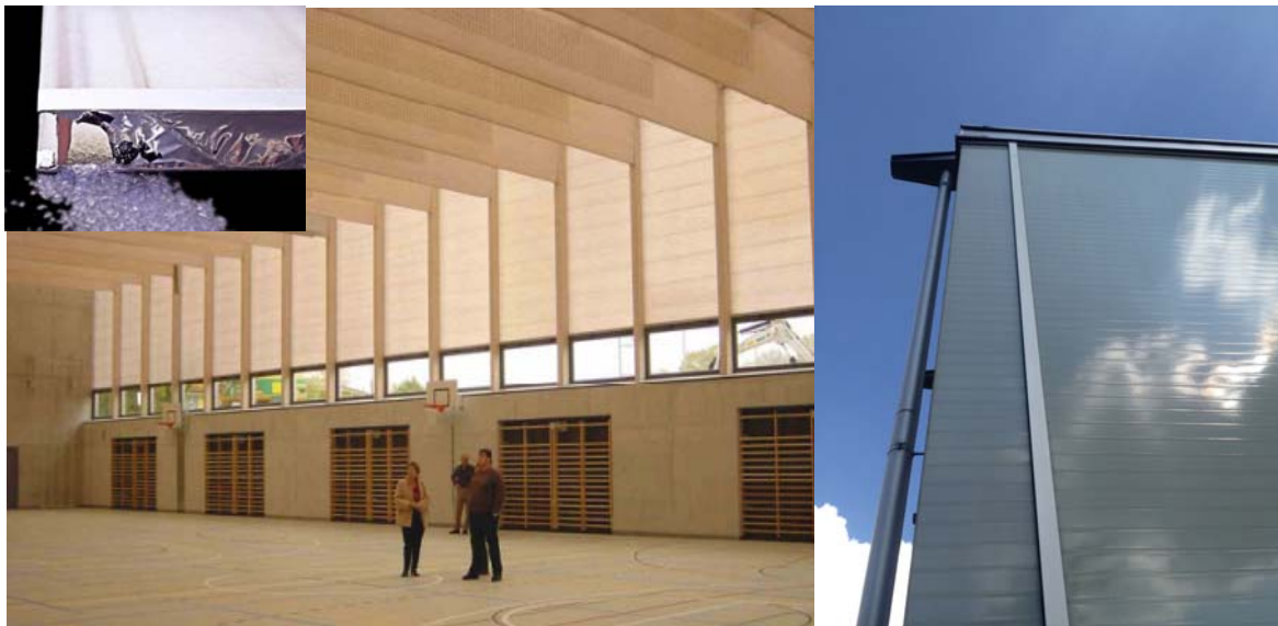
Figure 1: Translucent facade seen from the inner side in 2004 and the outer weathered façade photographed a decade later in October 2014. The inset visualises the granules which fill up the cavity and insulate.
