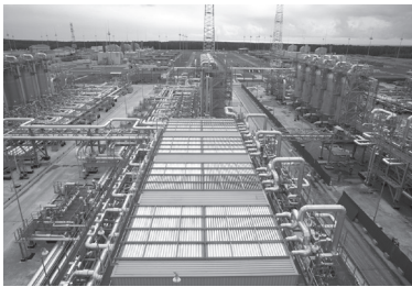
[69] Gas Treatment Unit Portovaya Bay, Russia.
