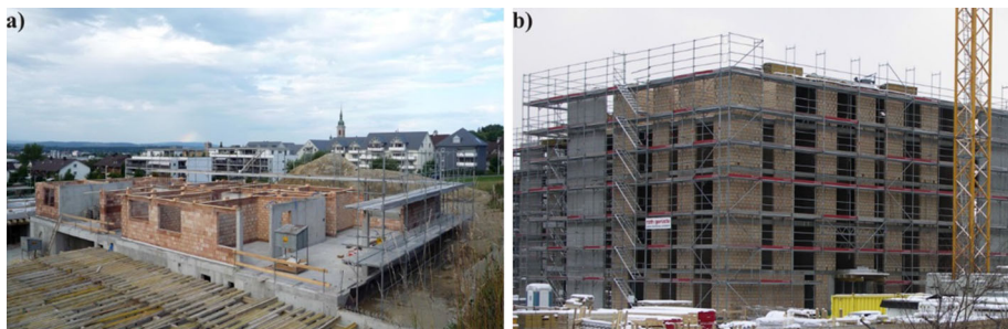
Fig. 1 Examples of new buildings with RC and URM walls in Switzerland (Photos: Thomas Wenk)
