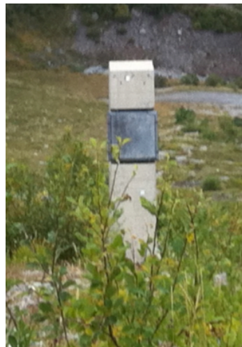
Fig. 2: The small concrete wall supports a 1x1 m 2 pressure plate.
