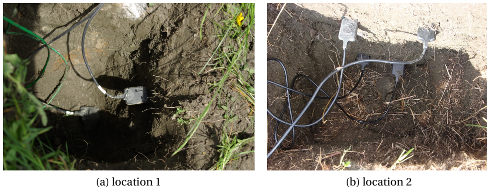
Figure 5.3: Installation of soil sensors at 20 cm and 40 cm at two different locations with different type of soil
