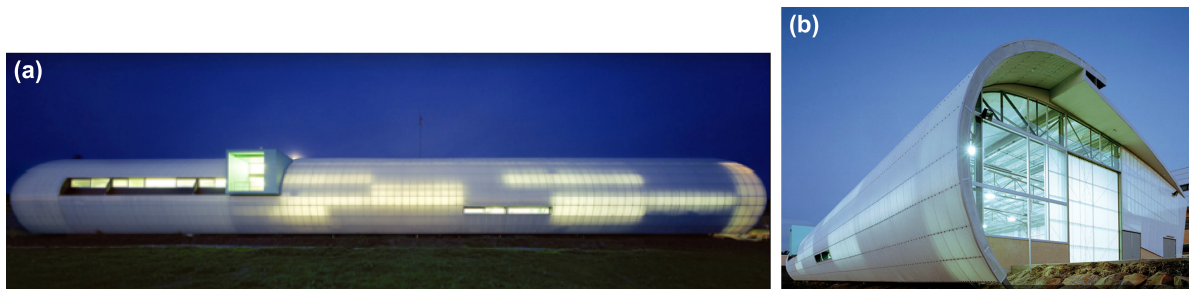
Figure 1.3. GFRP facade of Polymer Engineering Center from (a) front view at night and (b) lateral view (Melbourne, 2001).
