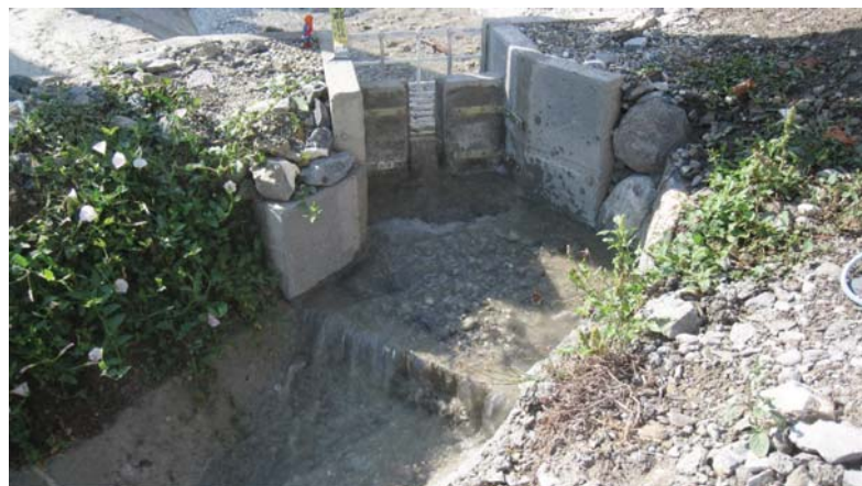
Figure 2. Physical model of the filtering dam with stilling basin, view from downstream.
