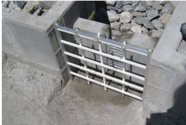
Figure 3. Floating debris screen installed in the physical model.
