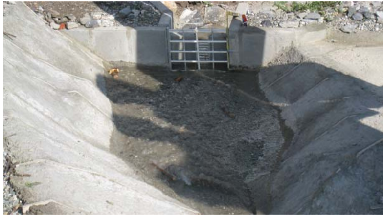
Figure 1. Physical model of the filtering dam with retention zone, view from upstream.
