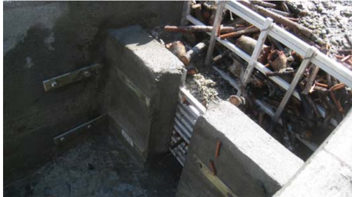
Figure 11. Situation at the dam after 100-year return period flood event on the physical model.
