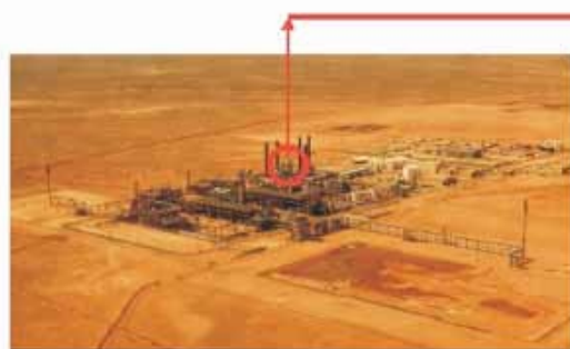
At In Salah, Algeria, natural gas purification by CO 2 removal plus CO 2 pressurization for nearby injection
