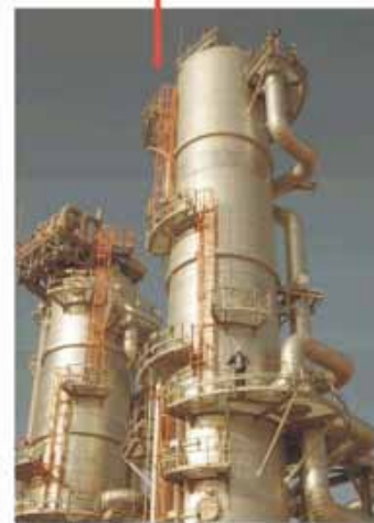
Separation at amine contactor towers
