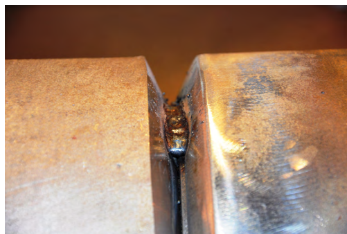
(d) Close-up of weld gap before tack welds being ground.
