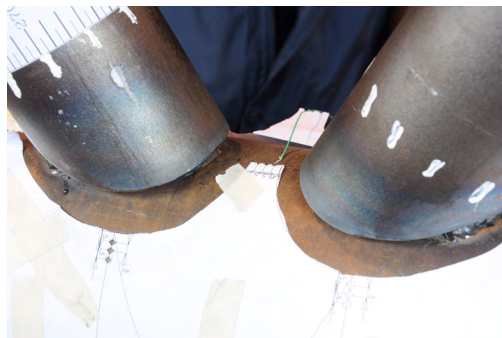
(c) K-joint before welding.
