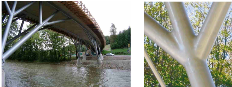
Figure 1.1: Traunstein (tree buttress) bridge with the detail of a cast node. Design R. J. Dietrich (Nussbaumer et al., 2010).
