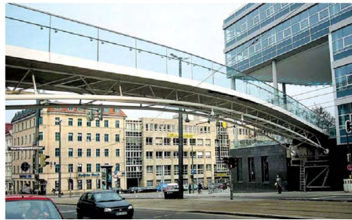
(b) Kurt-Heartel-Passage footbridge in Munich
