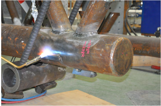
(a) Preheating the chord before welding of stopper piece.
