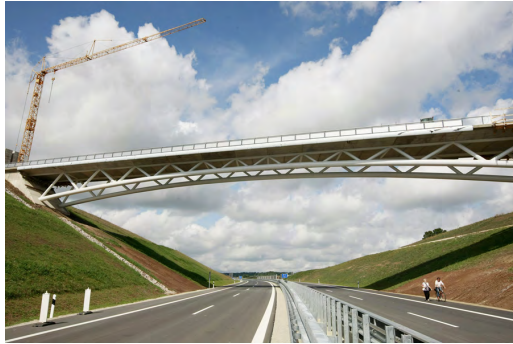
(a) Lichtenfels road bridge (span: 90.8 m)
