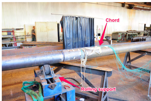
(c) Chord on the rolling jig for complete welding.
