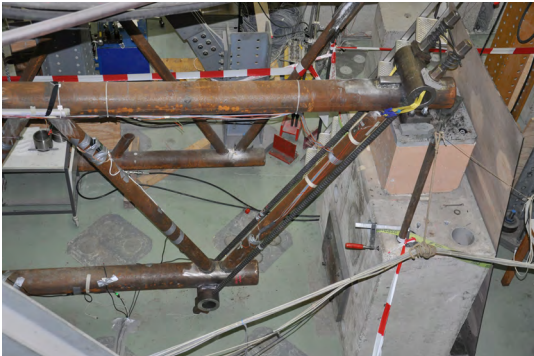
(d) Repair assembly fully mounted on truss.
