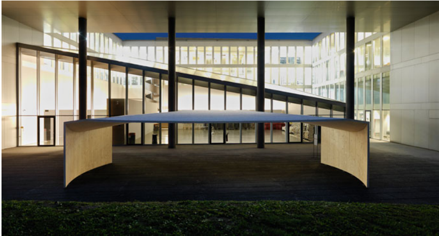
Fig. 1 Full-scale, mono-material prototype structure, spanning 13.5 m at a shell thickness of 77 mm, exhibited at the academy of architecture in Mendrisio, Switzerland
