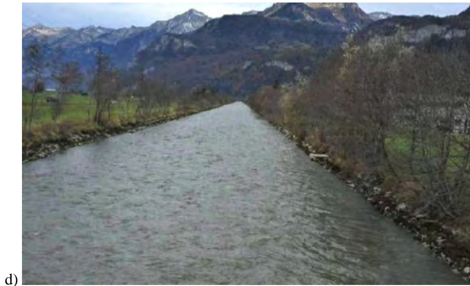
Figure 1.4: Picture of the Hasliaare River with (a) the minimum flow reach in Innertkirchen and the three types of engineered morphologies in the hydropeaking reach: (b) the groyne, (c) the gravel bars and (d) the channel (picture from Reto Haas) reaches. These reference reaches were used to model fish habitat. (All pictures were taken between October and November).
