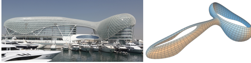
Fig. 1: Panel layouts can be represented by polygonal meshes subject to geometric constraints. Left: Yas Viceroy Hotel in Abu Dhabi, designed by Asymptote Architecture (image courtesy of Asymptote Architecture). Right: a quad mesh representing the hotel facade, with the constraint that the vertices of each face lie on a common plane. This constrained mesh represents a layout of planar quadrilateral panels on the facade.
