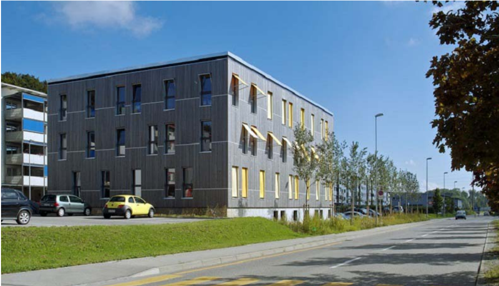
Figure 10: Green Offices Givisez, Switzerland
