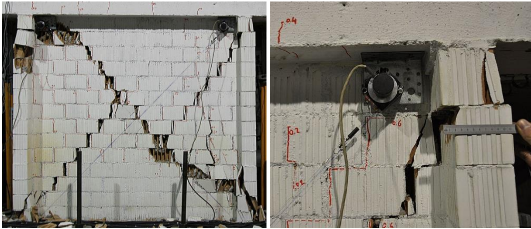
Figure 8. Residual deformations of one URM piers after test number 9.
