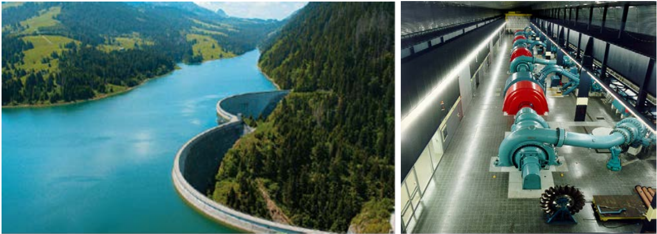
Figure 1: Hongrin Reservoir with the twin arch dam (left) and view of the existing 170 m long Veytaux 1 powerhouse (right) (source: www.alpiq.ch )
