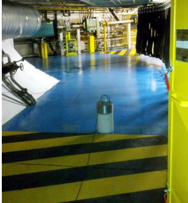
Figure 2 – The LUPIN placed in position 3, after the ventilation door.
