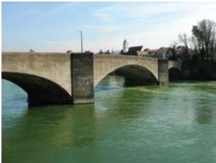
Figure 1. Historical concrete bridge over the Rhine river at Rheinfelden, designed and built by Robert Maillart in 1912.
