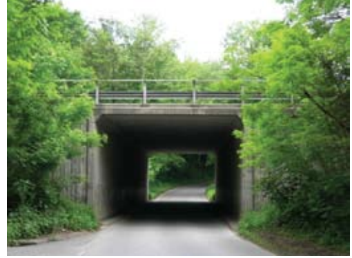
Figure 5. A: Underpass of a highway.
