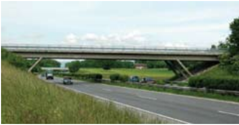
Figure 6. B: Overpass of a highway.
