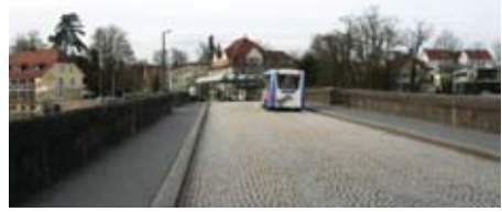
Figure 2. View of today's road lanes and pedestrian sidewalks.
