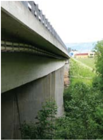
Figure 7. C: Highway viaduct.
