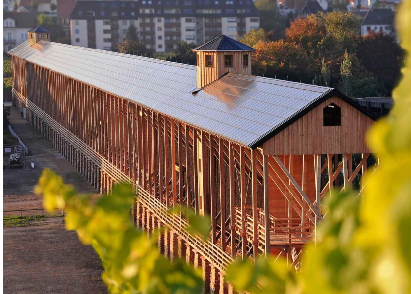
Figure 2: The saline of Bad Dürkheim in Germany is a very good example where the combination of photovoltaic modules (here thin silicon films modules) and historic building has been done harmoniously.
