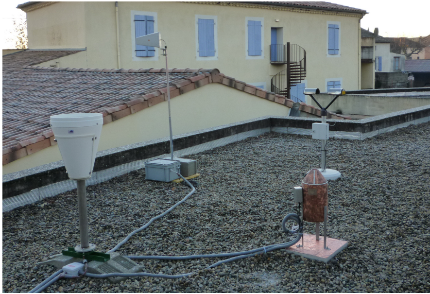
Figure 6.2: Example of experimental setup during the HPicoNet campaign on the roof of a school in Lavilledieu, Ardèche, France. The setup consists of a 1000 cm 2 tipping-bucket rain gauge (left), an optical disdrometer Parsivel (back-right) and an induction ring (front-right).
