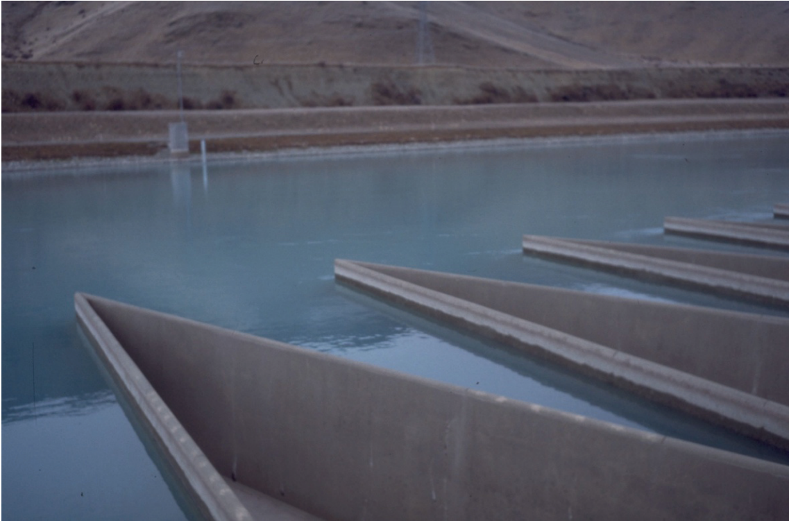
Figure 4 Triangular labyrinth weir of the hydroelectric power plant Ohau C in New Zealand.
