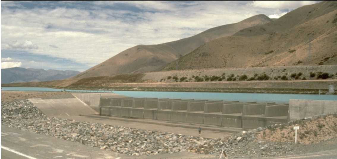
Figure 3 Labyrinth weir at Ohau river in New Zealand at the connecting canal between Ohau B and Ohau C hydroelectric power plant.
