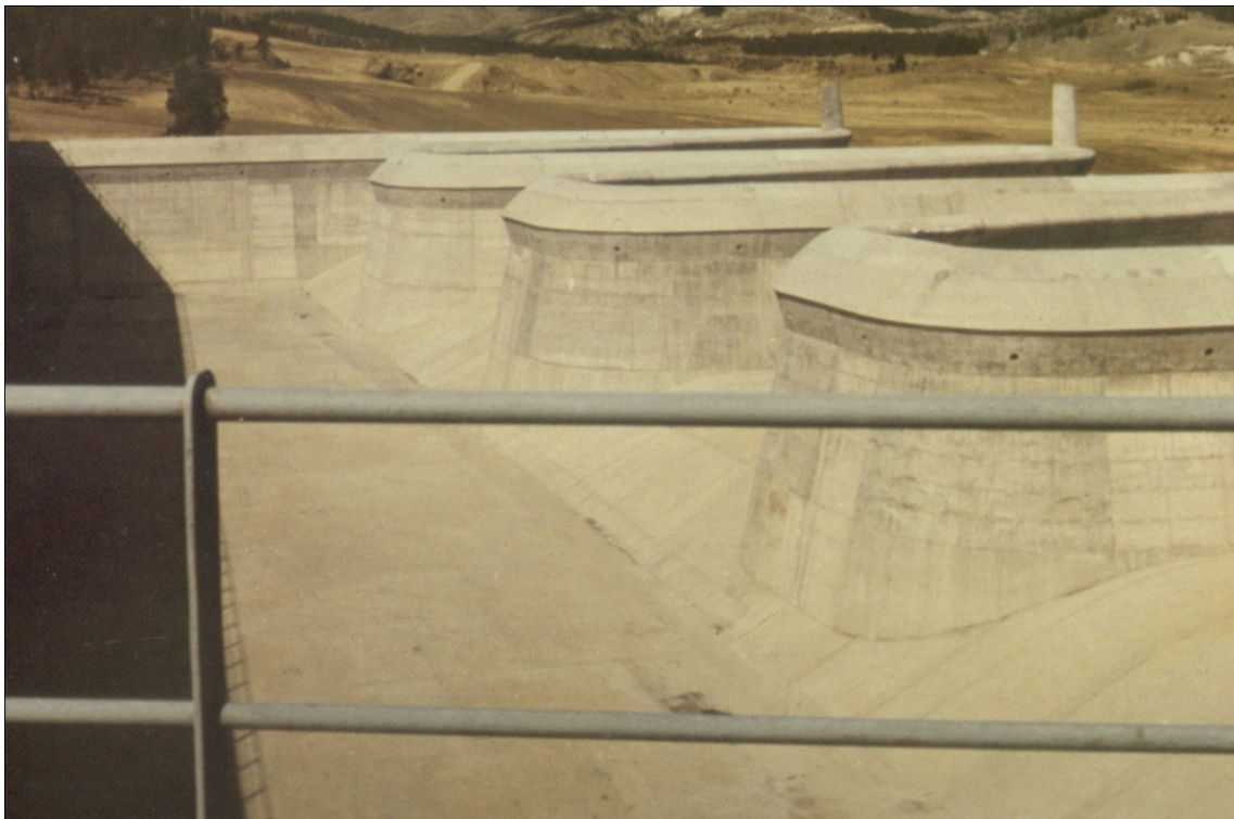
Figure 5 Trapezoidal labyrinth weir of Cimia dam in Italy.
