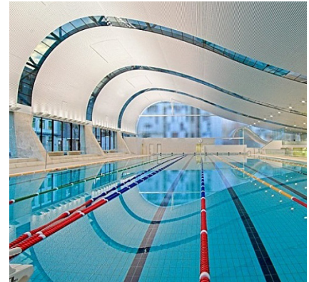
Example of artificial lighting on ceiling (Swimming Center, Sydney)
