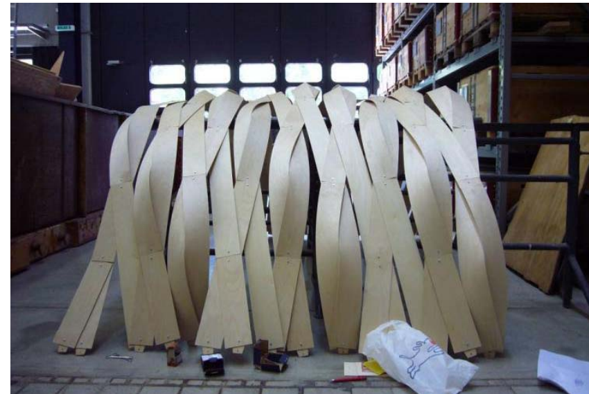
Timberfabric, interconnected elements, continuity in two directions;
